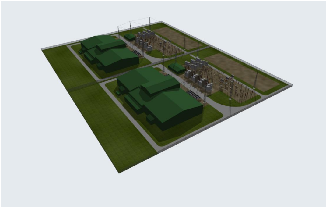
Plate 3 Indicative onshore project substation layout – HVDC
